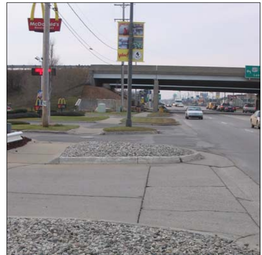
Multiple driveways on Pickard just east of US-127 lead to a variety of commercial uses.
